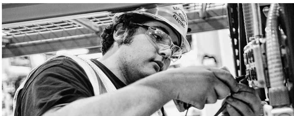
Anthony Sanchez uses a multimeter to test that wires are properly connected. He is an apprentice electrician with Esposito Electric, a 30-year-old Morris County business.
